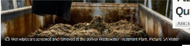
Wet wipes are screened and removed at the Usher Wastewater Treatment Plant. Picture: SA Water
